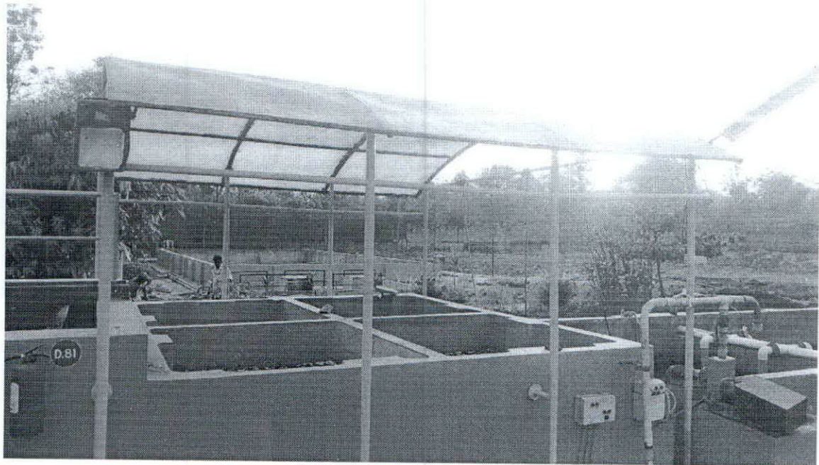
Fig 1.8 Oxidation Ponds
