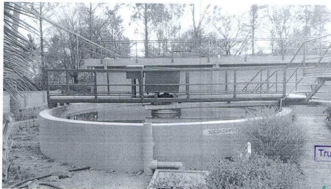
Fig 1.5 Secondary Clarifier
